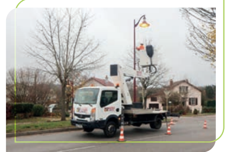
Installation des illuminations
